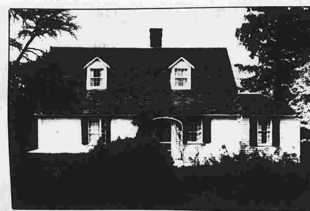
The best-known among the twelve homes that will be featured on the Manchester's Historical Society's calendar, the Cheney Homestead on Hartford Road was built around 1785. It serves as the society's headquarters.
