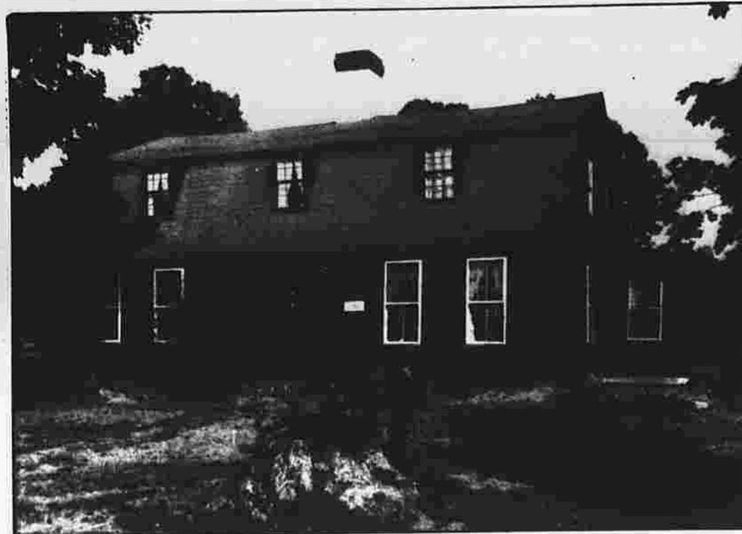
Believed to be Manchester's oldest standing house, the Brown House on South Main Street was built around 1752. For its first 30 years, the people that lived in the Dutch Colonial were still considered British subjects.
